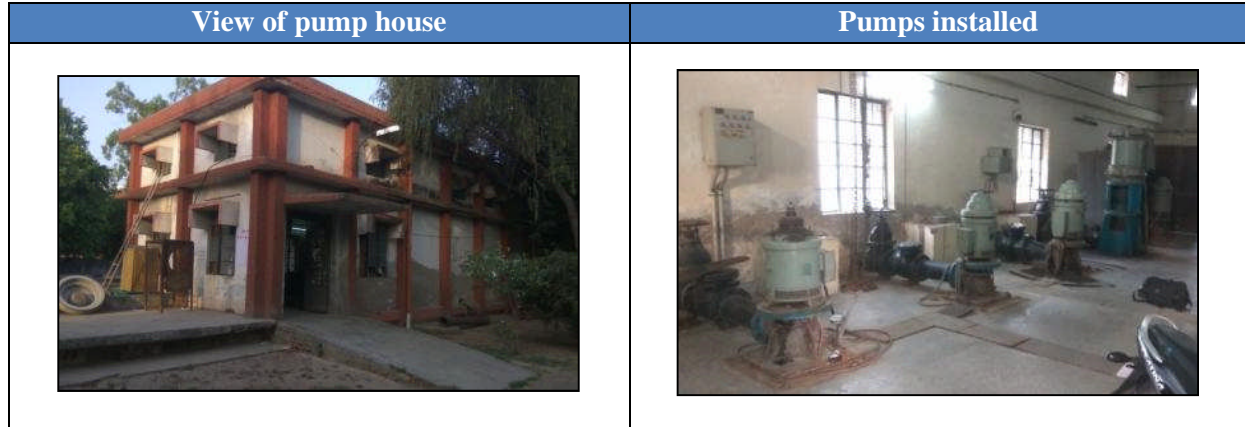
Figure 128: Photographs of Suryanagar ZPS
