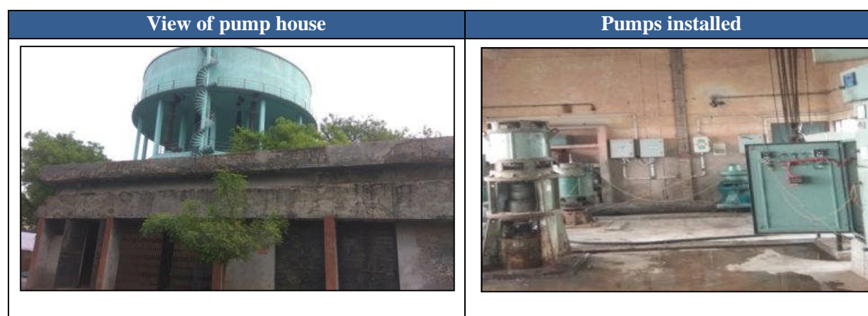
Figure 258: Photographs of Rakabganj ZPS
