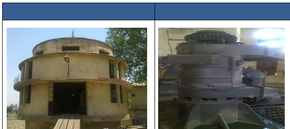
Figure 13: Photographs of Old Intake Well
