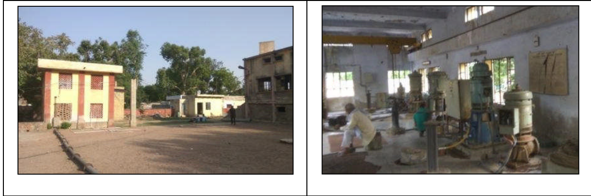
Figure 246: Photographs of Tajganj ZPS
